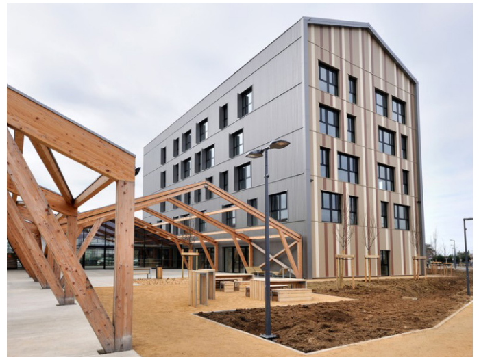
Figure 10 : Campus Formation SNCF – Saint Priest (69) | BBC Effinergie 2017 | Reichen et Robert & Associés | MO : SNCF
